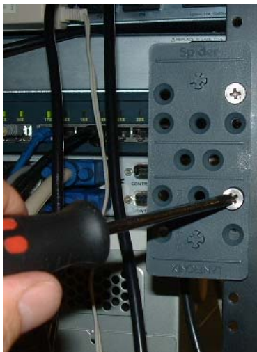
1. Mount the bracket with a Phillips-head screwdriver
