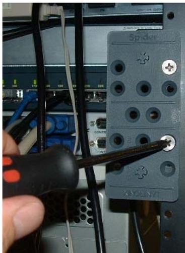
1. Mount the bracket with a Phillips-head screwdriver
