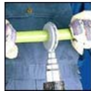
Butt-welding PVC
