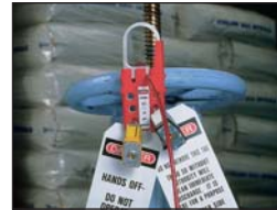
Lockout gate valves
