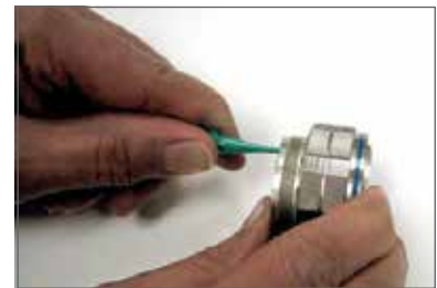
Plastic tool with contact in proper position.
