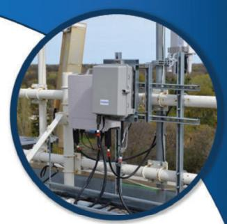
DC breakers enable the installer to switch off any single RRH during installation or mainte-nance operation without having to access the power supply rack usually located on the ground.
