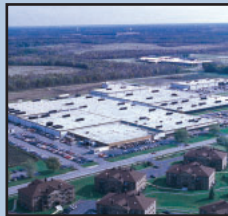
PANDUIT Corp. Worldwide Headquarters Tinley Park, Illinois 60477-3091
