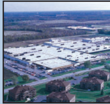
PANDUIT Corp. Worldwide Headquarters Tinley Park, Illinois 60477-3091
