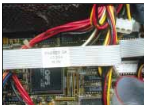
Flat Ribbon Cable Labeling
