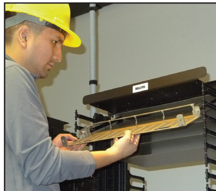
Slide-in trays tilt outward to improve accessibility.
